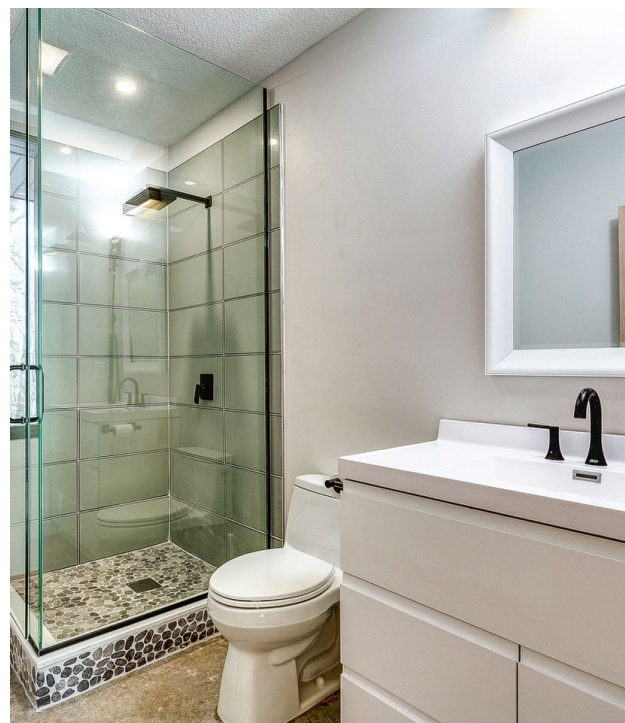
Green lavatory. Water-conserving fixtures—faucet, toilet, showerhead—as well as energy-saving LED and natural lighting, abound in the bathroom. CREDIT: COURTESY OF SIPA
