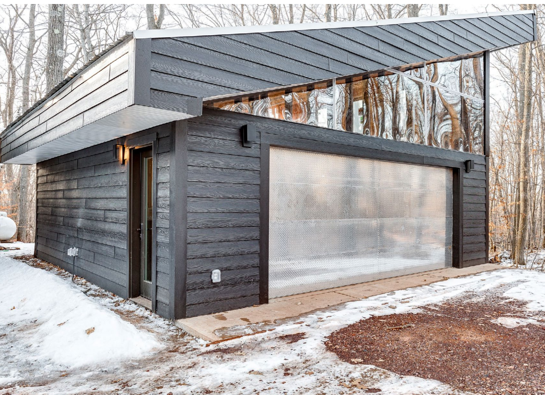
Right angle. A 5-foot overhang shades half of the home's south-facing windows in summer, but allows house-warming sunlight during winter thanks to its angled metallic roof. CREDIT: COURTESY OF SIPA
