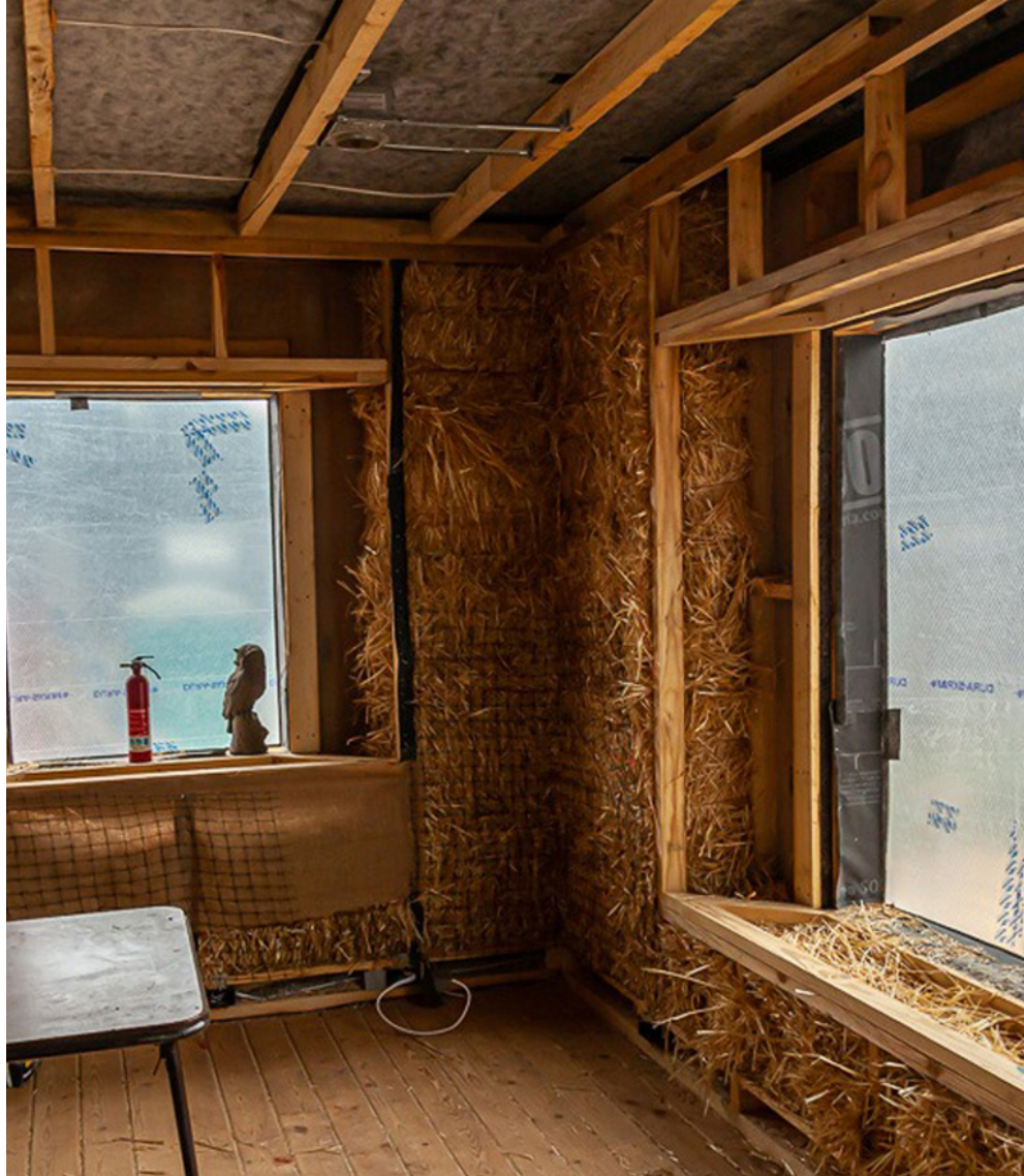
The last(ing) straw. A key component of Habitat for Humanity Gunnison Valley homes is straw bales, which are used as an all-natural and easily obtainable form of insulation. It's also highly fire resistant and, under the right circumstances, can last decades. PHOTO: HABITAT FOR HUMANITY GUNNISON VALLEY
