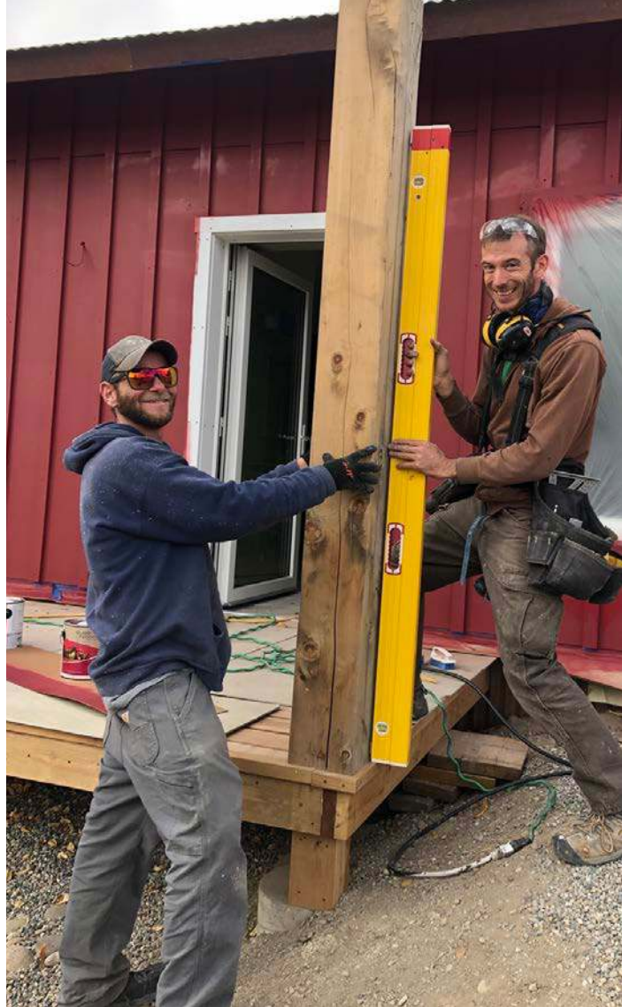
Joint effort. Volunteers with construction experience worked together to quickly build energy efficient Gunnison Valley homes.
