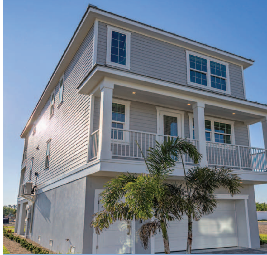
Above the bay. Hunters Point homes are three-story, with the bottom level serving as protection against flooding.
