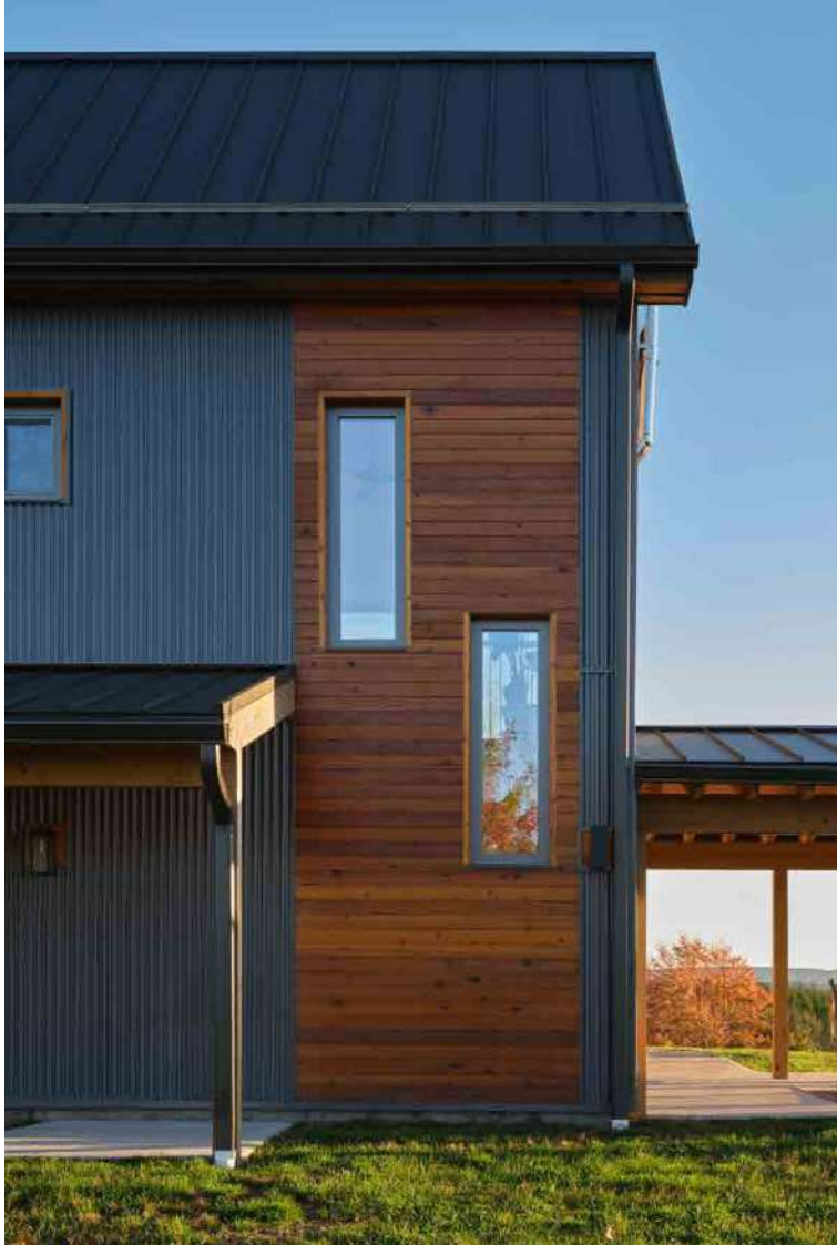
Glass housing. IKON triple-glazed windows let in light and heat from the low sun in the winter months, providing a natural form of indoor environmental control. CREDIT: FRAZIER SPRINGFIELD PHOTOGRAPHY
