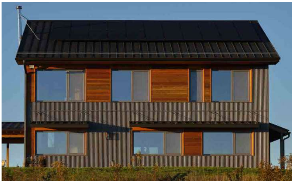
Less than zero. The Fairview Passive home produces more energy than it consumes thanks to an 8.8-kilowatt rooftop solar array. CREDIT: FRAZIER SPRINGFIELD PHOTOGRAPHY
