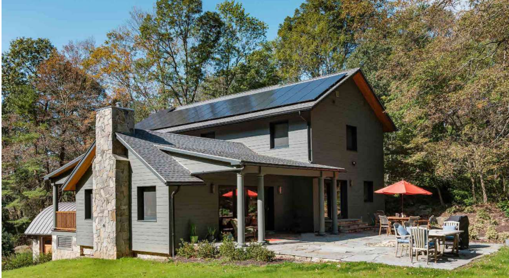
Sun sense. Utility electric service is supplemented by an 18-kilowatt roof-mounted solar photovoltaic array. CREDIT: MADDEN STUDIO/BRIAN A. MADDEN
