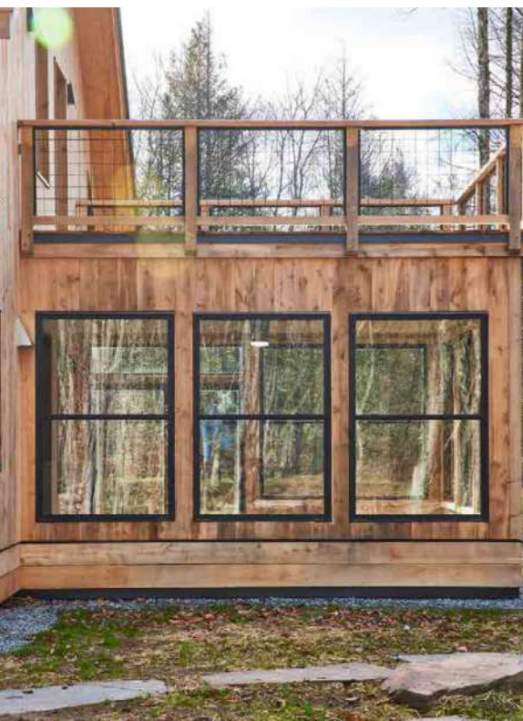
Sun block. Triple-pane aluminum glass windows help control sunlight and external heat. CREDIT: WOLVESTUDIOS/ADAM FITHERS
