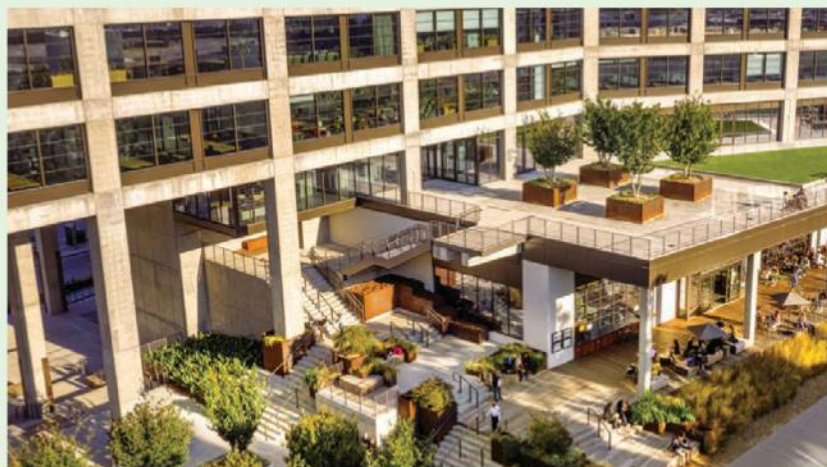
Structurally sound. The 725 Ponce building in Atlanta, made entirely with carbon-mineralized concrete, is one of CarbonCure's top achievements.
