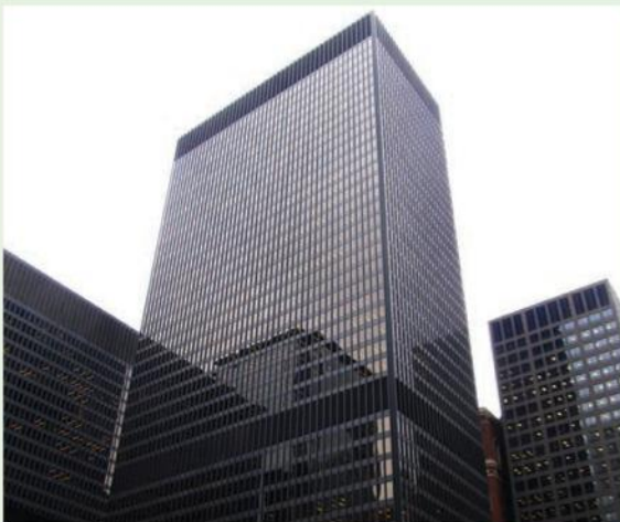
Federal facelift. After 40 years, the John C. Kluczynski Federal Building in downtown Chicago needed a sustainability upgrade, especially in its 78 bathrooms. COURTESY OF KEN LUND/FICKR
