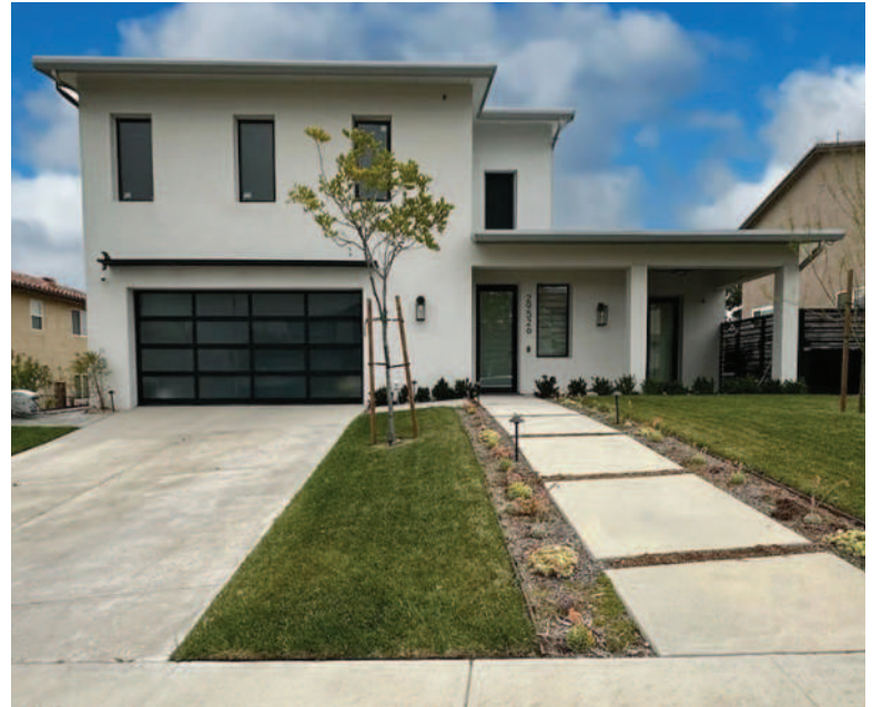
Hot topic. The PHNX Home , built in California's Santa Clarita Valley to replace a house destroyed in the 2019 Tick Fire, gives the homeowners greater peace of mind if such a wildfire should happen again. COURTESY OF PHNX DEVELOPMENT
