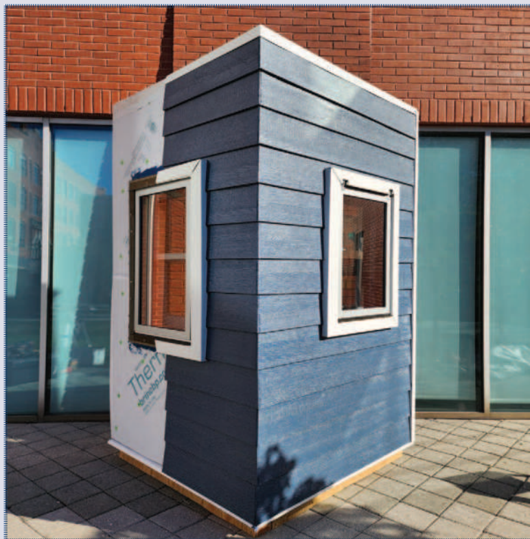
A better rebuild. The mock-ups consist of two inches of rigid insulation, liquid flashing, a thermally broken window surround, high-performance exterior storm windows, and new siding. CREDIT: COURTESY OF U.S. DEPARTMENT OF ENERGY
