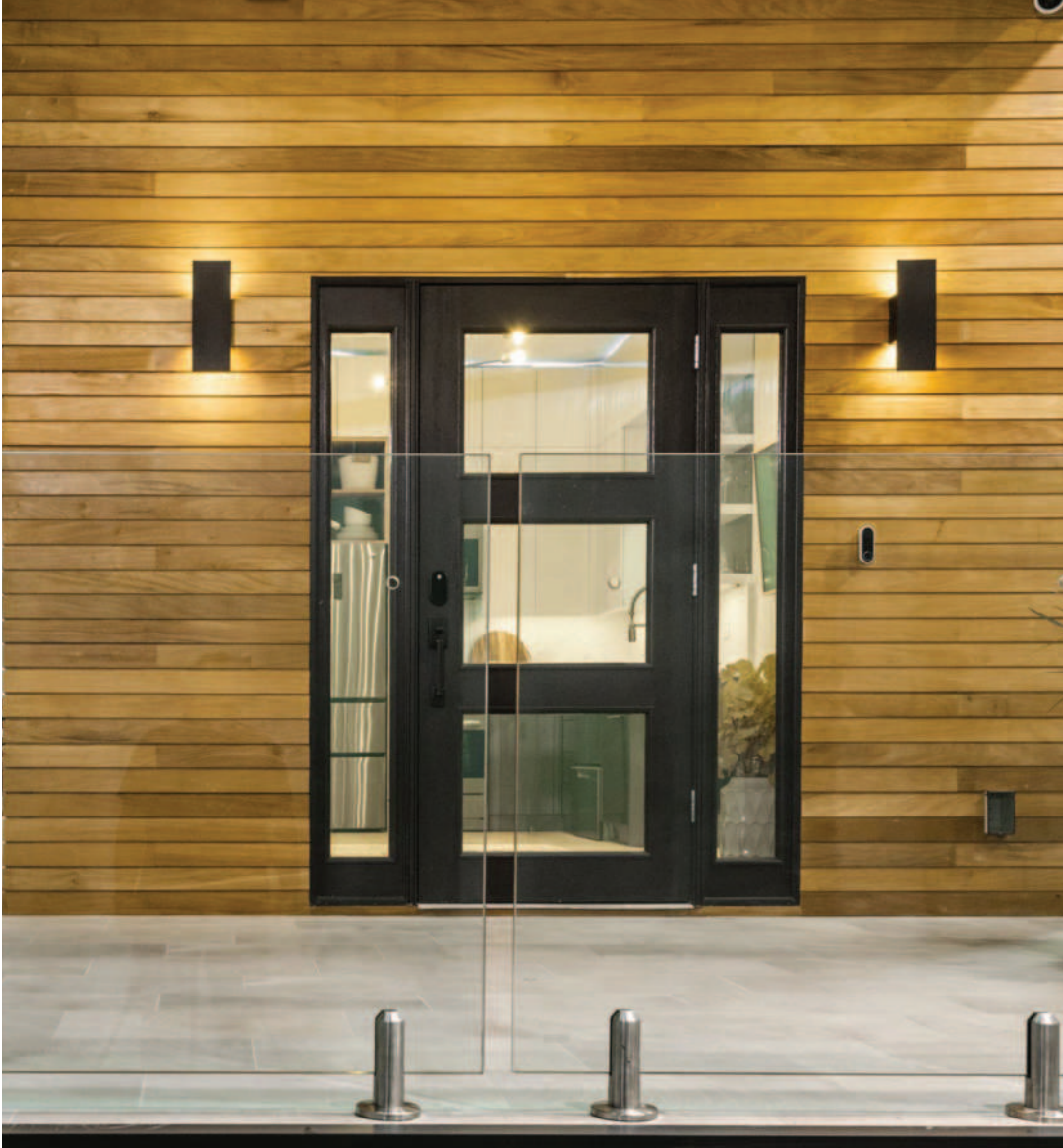
Built to last. Pearl Concept was built with sustainable materials, including steel, aluminum and timber, and included energy savers such as LED lighting. CREDIT: COURTESY OF PEARL HOMES
