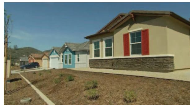
In the clear. Wildlife Prepared Home Plus certification and the California Department of Insurance require a noncombustible perimeter buffer and defensible space zone around each house. CREDIT: COURTESY OF KB HOME
