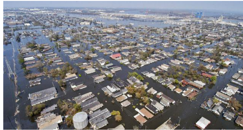
Not ready for nature's worst. Lackluster building codes are enhancing property damage seen by coastal cities, such as New Orleans, the victim of weather-induced flooding several times over the past decade. SOURCE: CAN EUROPE/FICKR
