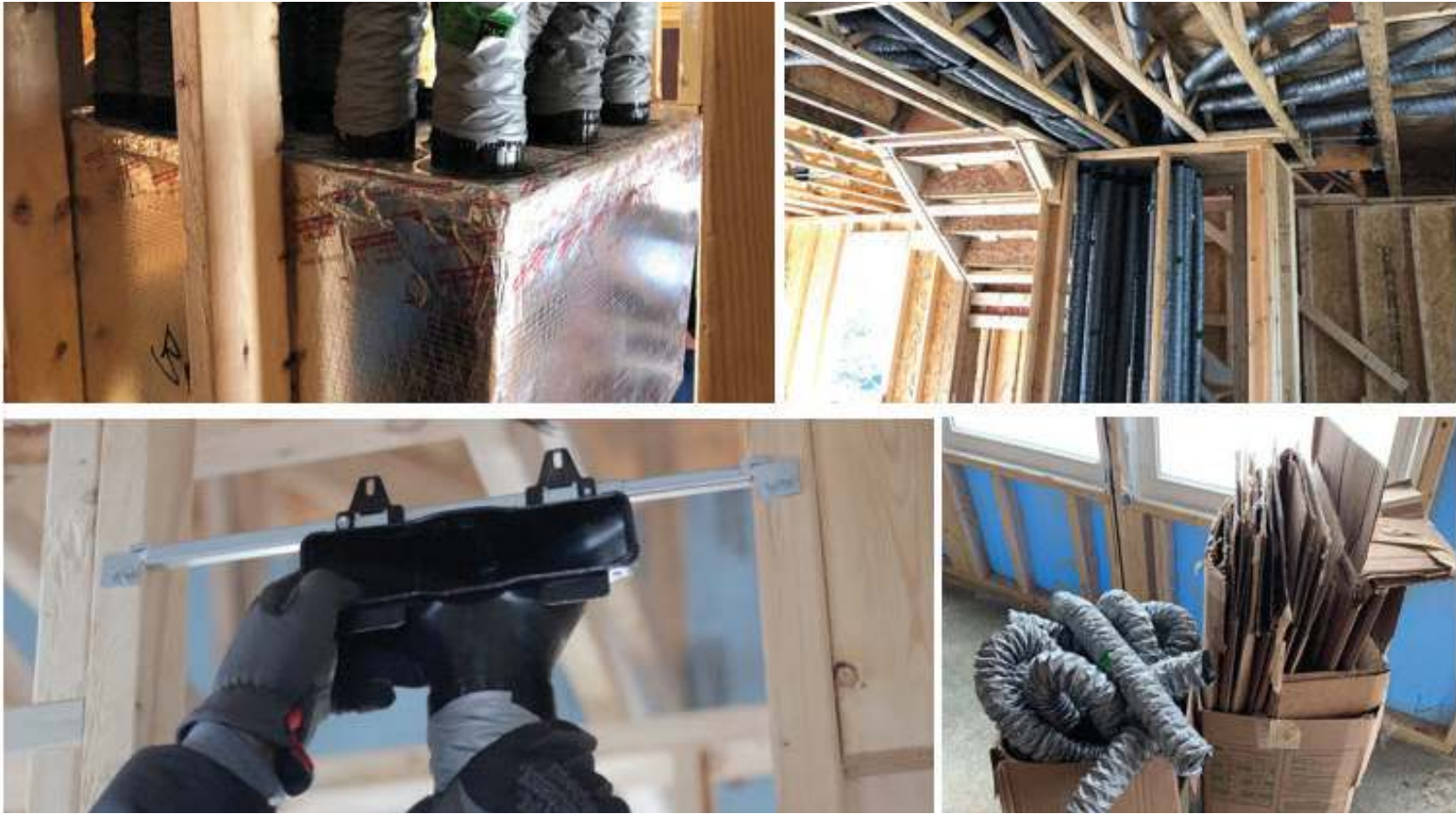
Figure 6: A plug-and-play duct system easily snaps together and is automatically airtight.
