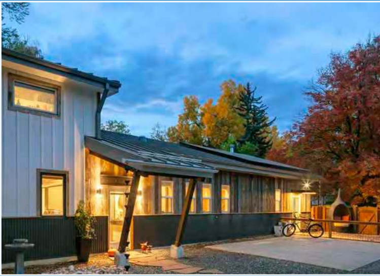
The old metal siding on the back section of the barn was replaced with reclaimed wood.
