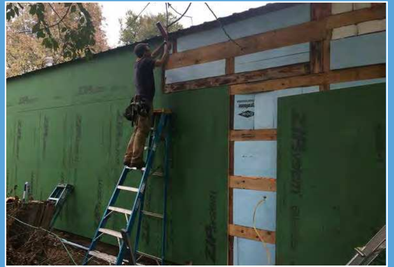
Exterior walls were removed and ZIP System R-sheathing rigid wrap was installed during the renovation of the barn, which had numerous gaps and cracks that contributed to an excessive ACH of 11.
