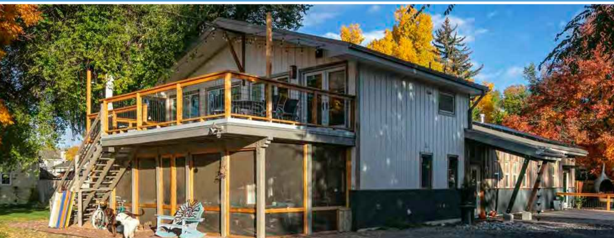
LEFT: Old double- and single-pane windows were replaced with new energy-efficient units.
