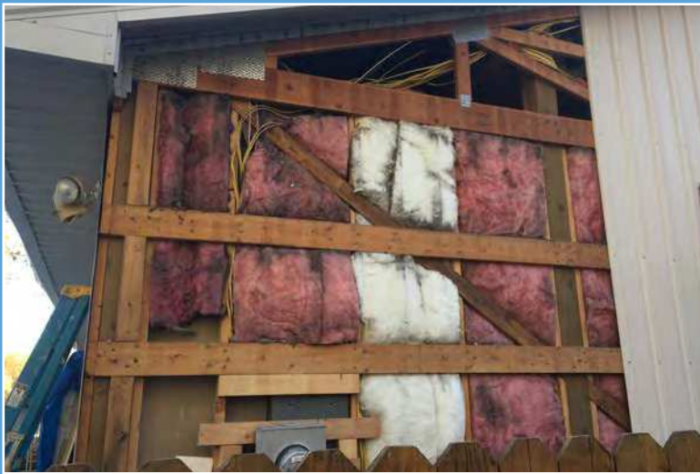
New and reused insulation were placed between the studs of the house to provide better sealing.
