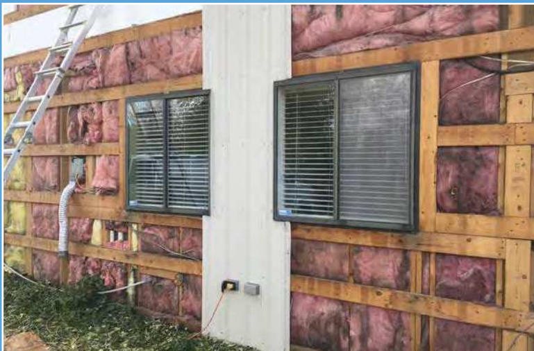
Leaky windows were replaced with energy-efficient units. Insulation from elsewhere in the house was reused wherever possible.
