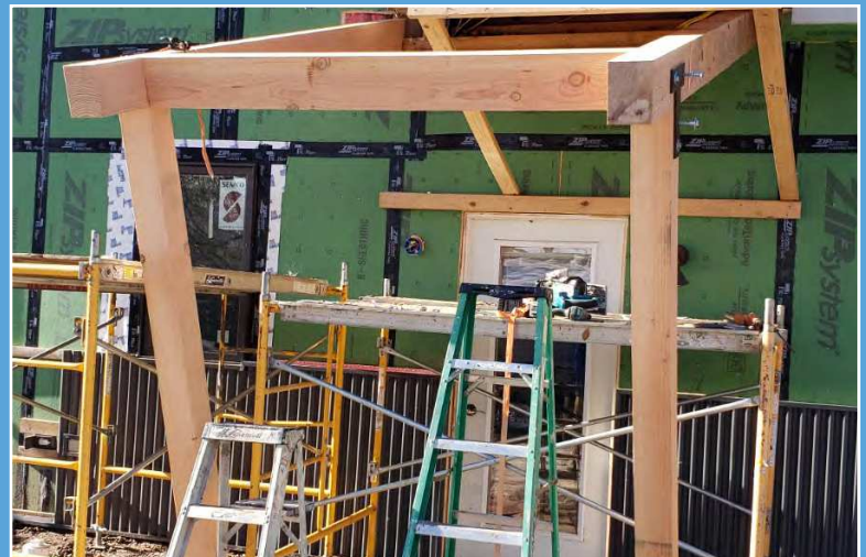
An overhang was added above the front door for aesthetics, and to keep snow and rain from the main entrance.
