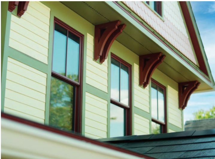
The Queen of Zero is a rebuilt historic home in the Washington, DC area featuring Hardie® products to deliver a historic Victorian design with a modern standard of resiliency and durability.
