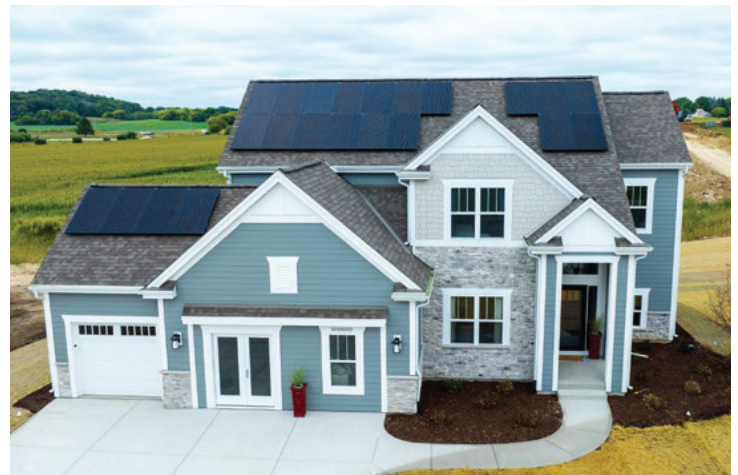
James Hardie joined award-winning builder, Tim O'Brien Homes, on a new construction, next generation home called VISION House Sussex to create an attainable green home for American families in the upper Midwest, featuring Hardie® siding.
