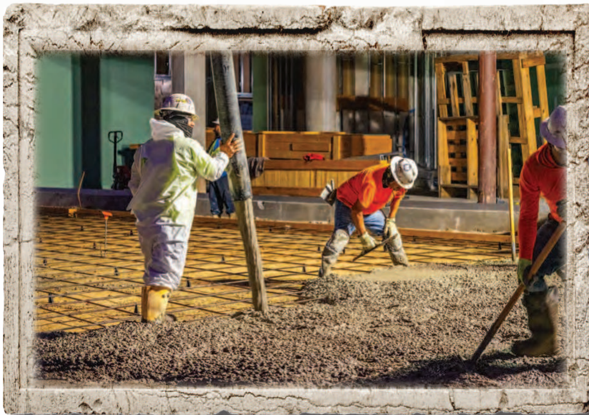
Equal footing. Recycled or “green” cement—such as Terra CO2 Technologies’ waste granite-developed OPUS SCM at a project in Sugarland, Texas—provides a surface that is environmentally friendlier but just as durable. CREDIT: TERRA CO2 TECHNOLOGIES
