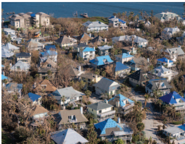
Weather resistant. Some homes went through Hurricane Ian without any problems outside of a heavy storm. Otherwise, life goes on as usual. COURTESY OF SOUTH FLORIDA WATER MANAGEMENT DISTRICT
