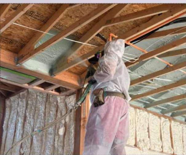
Twice the benefit. To conserve energy, the Forever House features roofing with R-70 insulation, a product that is 22-25 inches thick—about 1 foot more than the R-38 used on most homes in the area. PHOTO COURTESY OF STEVE EASLEY
