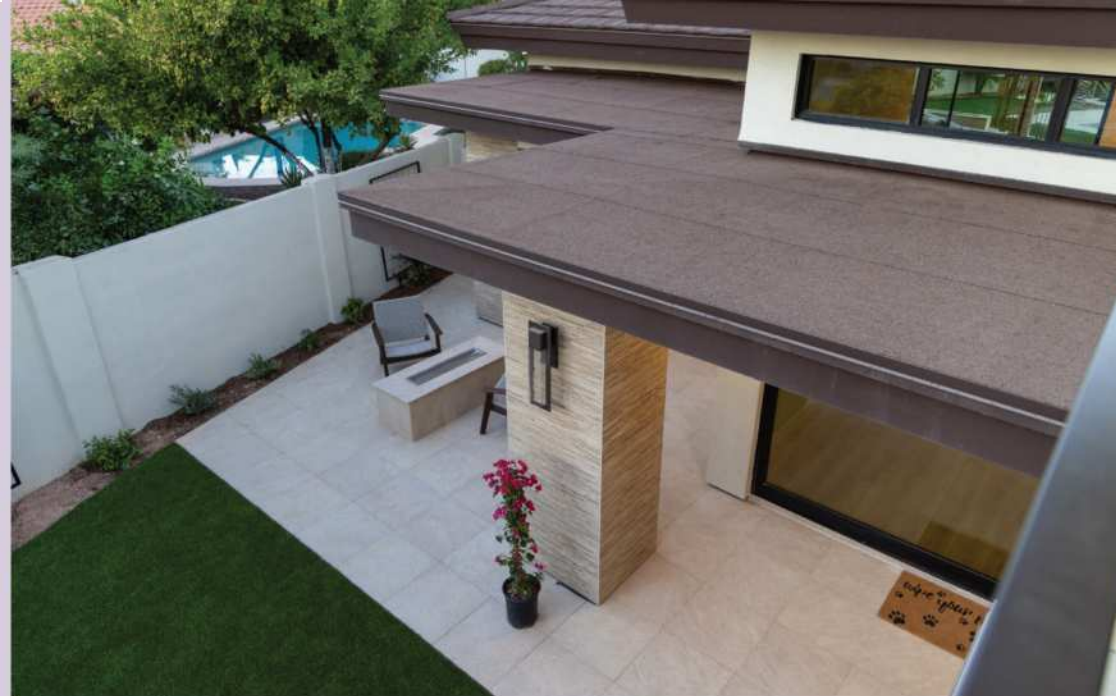
Under cover. The home's passive design included large porches with overhangs on the south and west sides of the house to reduce heat exposure in the summer. PHOTOS (left and right) BY SAMANTHA CARLIN/GREEN BUILDER MEDIA
