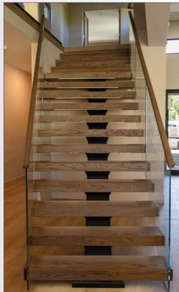
Stepping up. The stairs are a mono stringer floating stair case from ViewRail. The stair system was prefabricated offsite and installed efficiently onsite.
