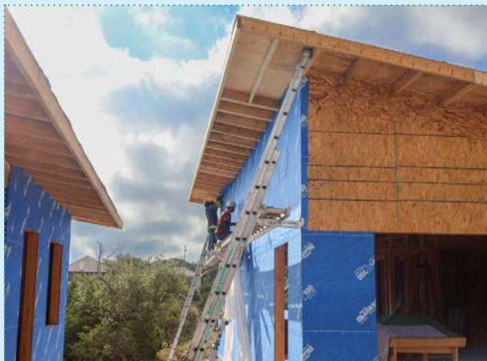
A tight situation. Insulation from Henry Company helps protect the VISION House Austin and the garage from water, air and moisture intrusion.
