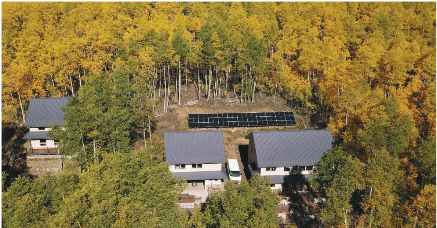
Grid be gone. Mariposa Meadows utilizes a solar array, battery storage system and backup generator to meet its electrical needs.
