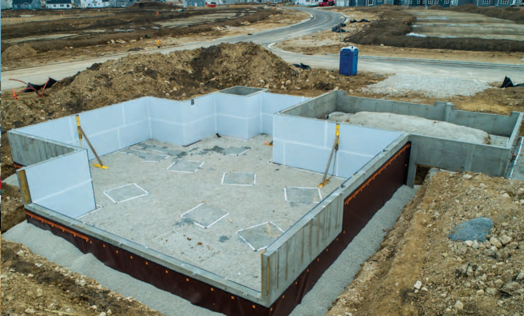
Rock solid. Eight-inch-thick concrete slabs distribute the weight of the home and prevent water seepage. COURTESY OF TIM O'BRIEN HOMES
