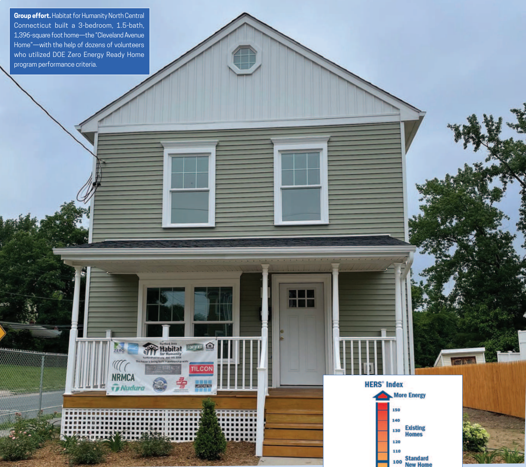
PHOTOS COURTESY OF HABITAT FOR HUMANITY NORTH CENTRAL CONNECTICUT
