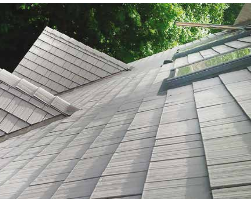
New old-fashioned look. Enviroshake's composite tile combines the feel-good nature of wood with the long-term durability of clay.
